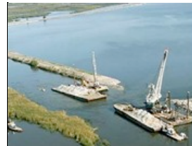
Jones Tract levee during it's construction. (File) Dept. Of Water Resources
